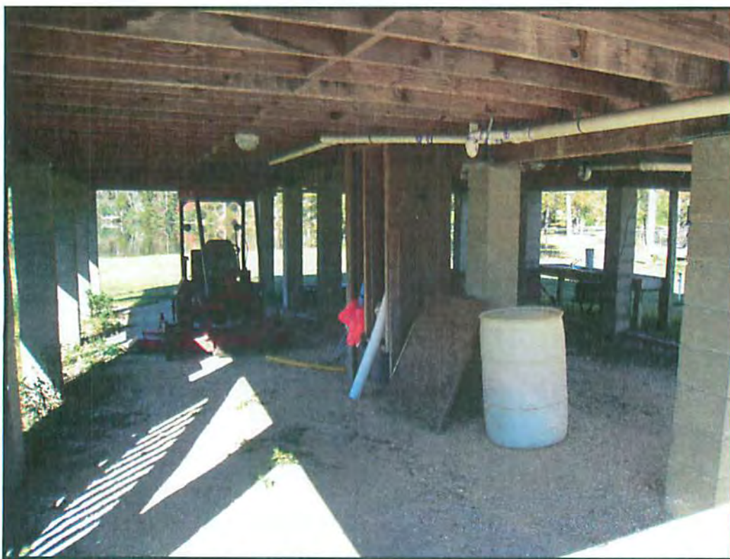
VIEW OF GROUND LEVEL PARKING/STORAGE AREA BELOW STRUCTURE
