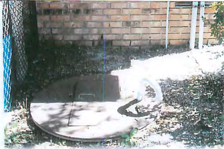
Sanitary sewer connection – 1505 W. Avery Street, Beulah's Pre-K
