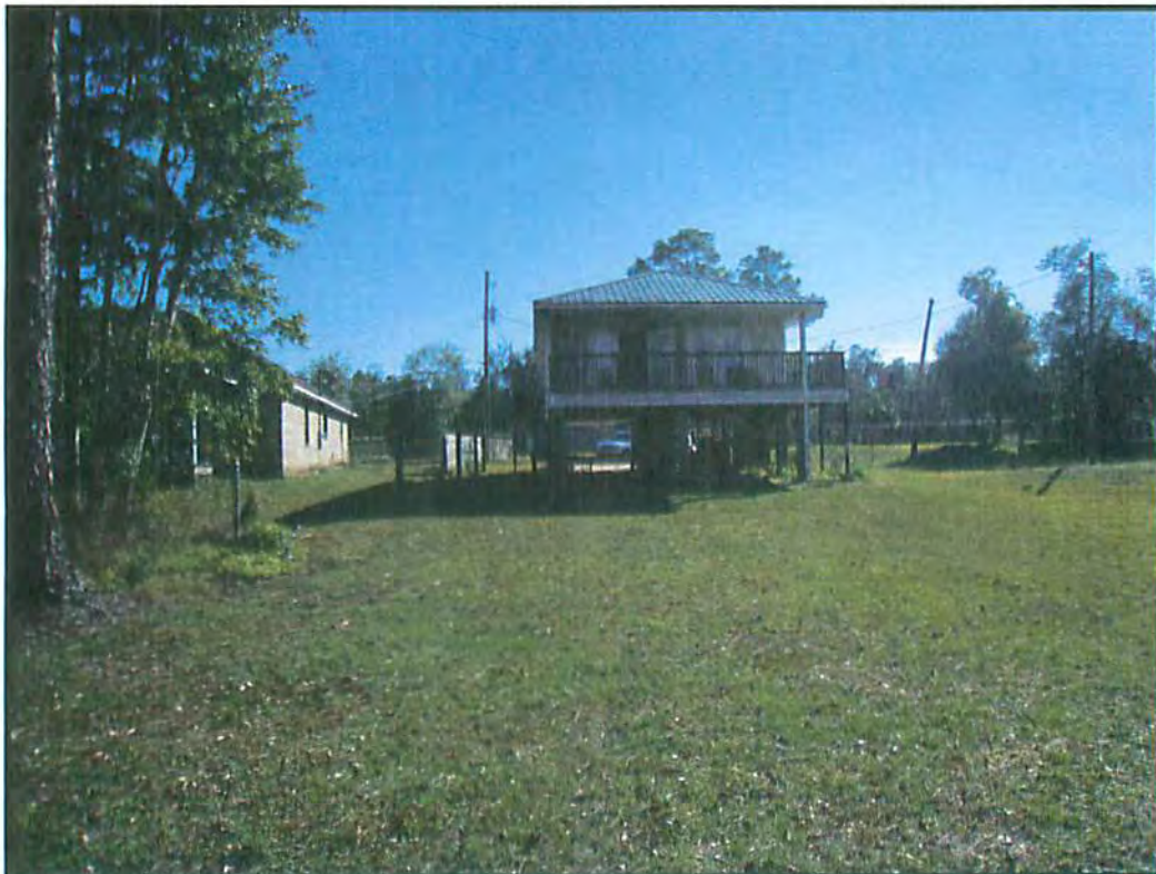
SOUTHERLY VIEW OF PROPERTY – TAKEN NEAR RIVER FRONTAGE
