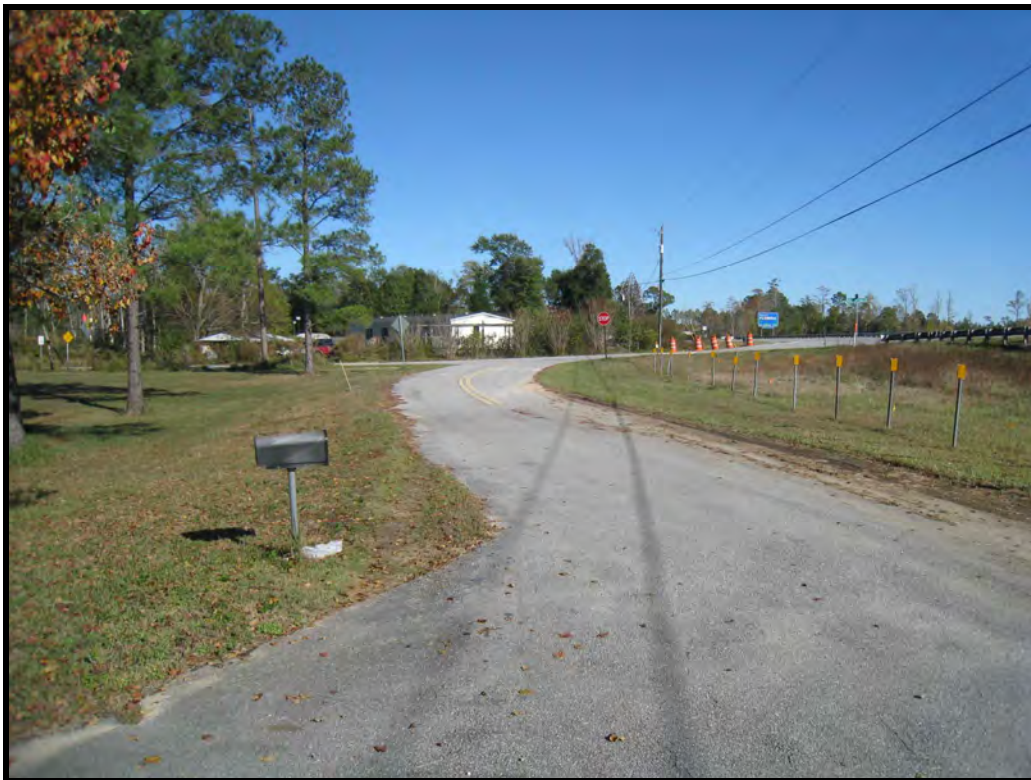
EASTERLY VIEW ALONG SERVICE ROAD FOR MOBILE HIGHWAY
