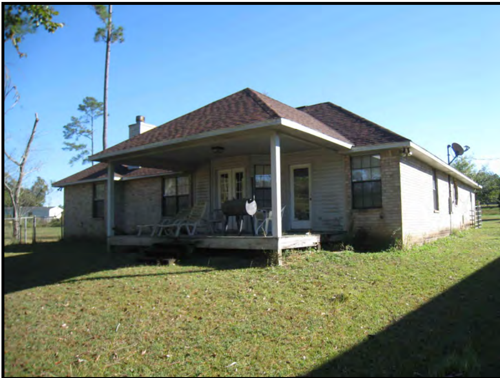
SOUTHEASTERLY VIEW TO REAR OF RESIDENCE
