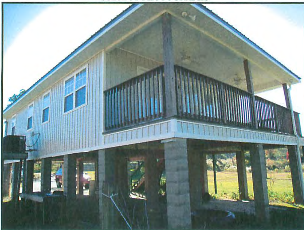
SOUTHWESTERLY VIEW TO REAR/SIDE OF RESIDENCE
