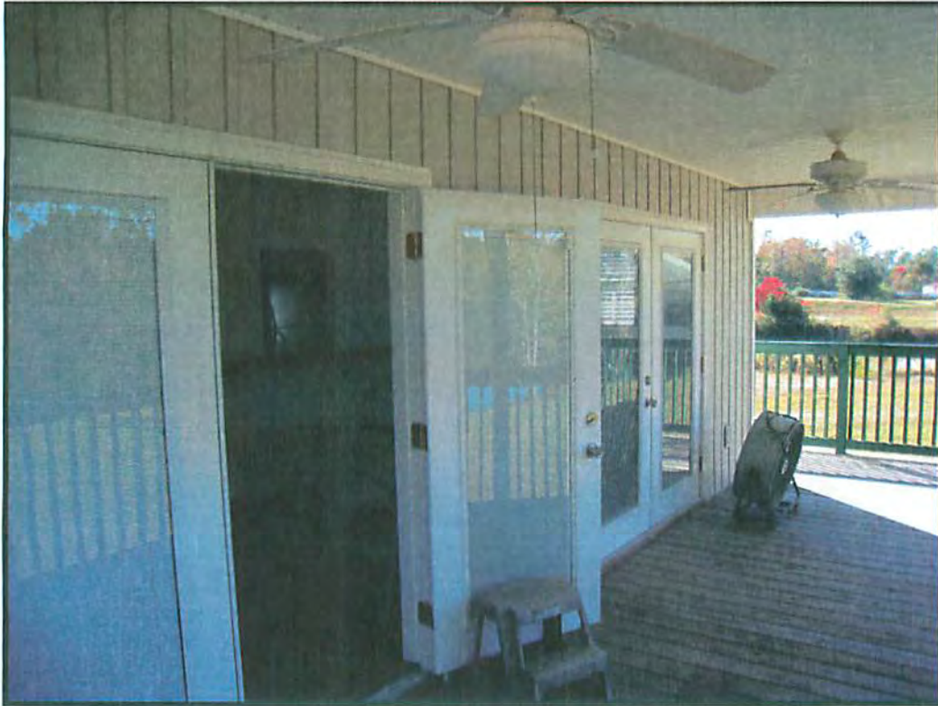
VIEW OF COVERED BALCONY
